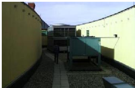
Equipment hidden on roof behind parapet wall
