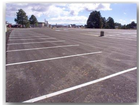
Parking lots with little amount of landscaping are discouraged
